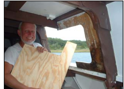
A bothersome window leak turned out to require replacing a whole section of wall
